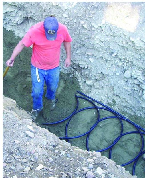
Figure 3 Slinky loop installation.
